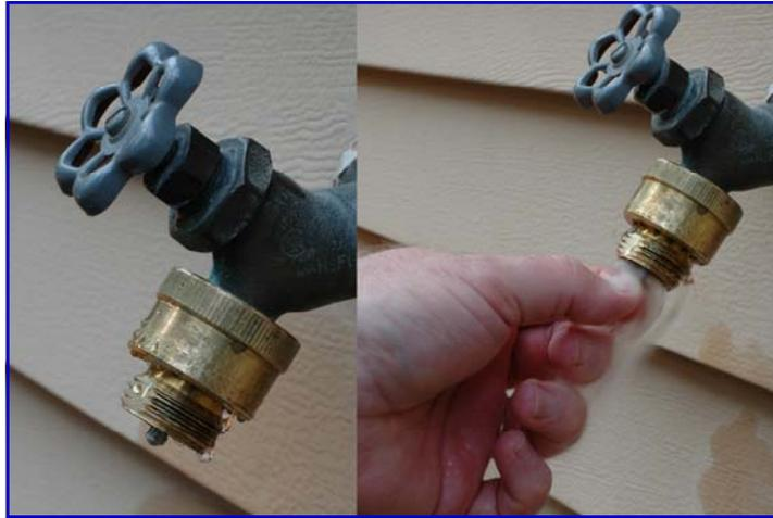
Be sure to open anti-siphon devices, if installed, to fully drain lines.
